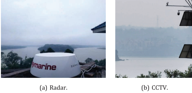
Fig. 9. Installation sites of radar and camera.
