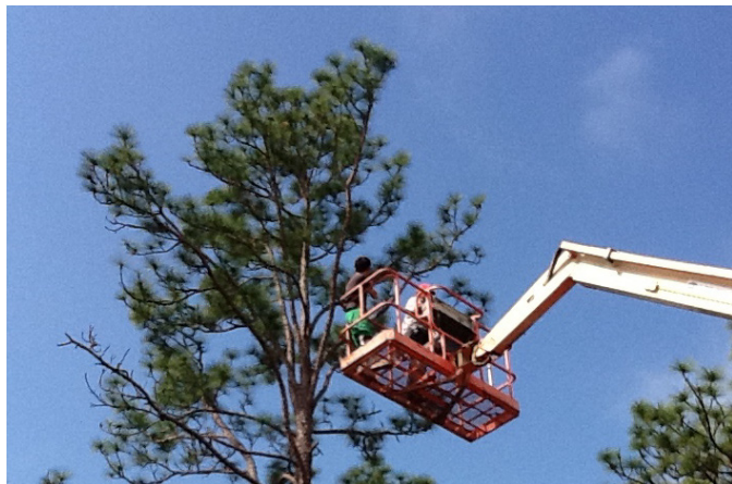
Fig. 12. Emplacing a high gain 13 dBi Yagi 1.3 GHz antenna in a tree at 25 m AGL using the bucket loader.
